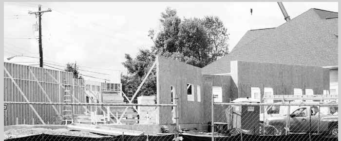
Progress at the addition to MCCH's Men's Emergency Shelter.
