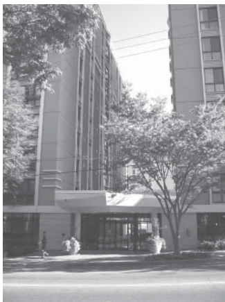
A condominium complex formerly homeless individuals now call home.
